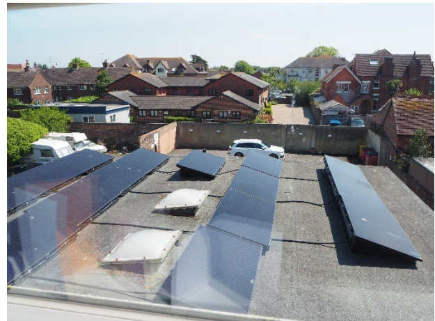
The arrangement of solar panels.
