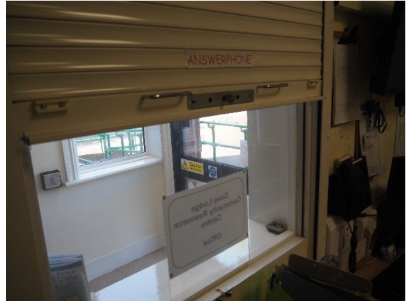
View of fire / security shutter.
