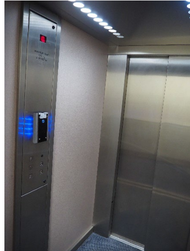
The inside of the lift car.
