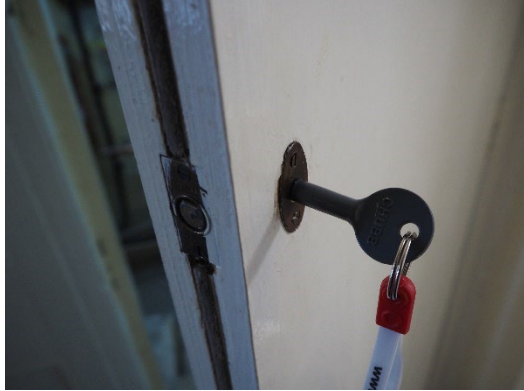
The door to the understairs storage cupboard.
