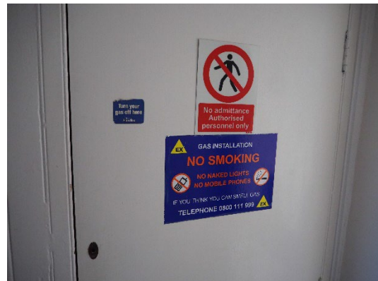
Door to services cupboard.
